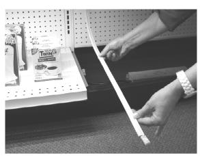
Step 3: From the base slide the track up behind the shelves; cut to fit length of uprite if needed Use scissors or similar cutting tool DO NOT cut the end with the yellow connector!
